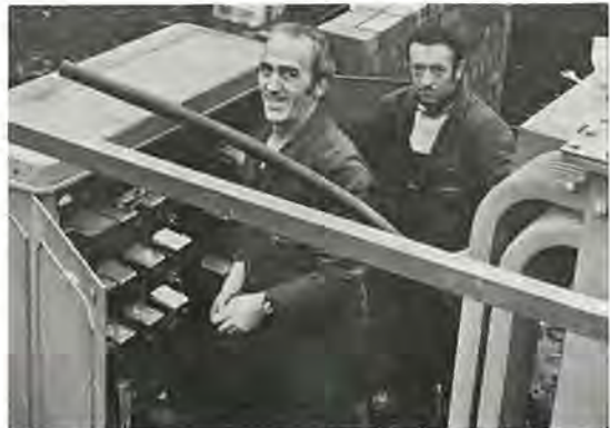
In the new compound substation established on site are members of the engineering staff, Jack Devaney ( ehv joiner ), left, and Derrick Parry ( joiner's mate ).
