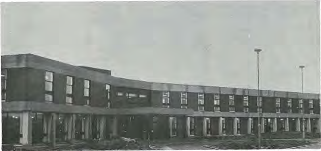
After waiting patiently for the sun to shine, we finally had to be satisfied with this picture of our new District Office block at Cefndy Road, taken in the pouring rain!
