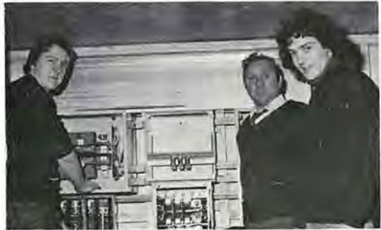
Working on the hastily constructed switch panel, from left to right: Steve Jones (apprentice), Eifion Jones (chargehand) and Emyr Williams (electrician).
