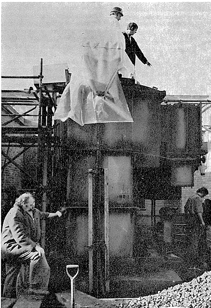
The replacement 35-ton transformer in its new bay. In the left foreground is Mr. Jack Critchley from Production Control at Head Office.
